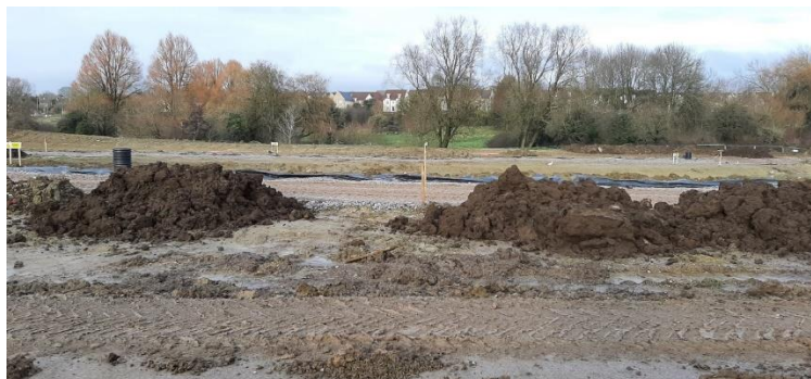
Cycle track under construction
